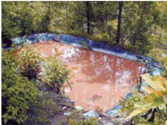
Picture left: Example of water reservoir/ pond, made by excavation and plastic sheeting to prevent leakage. Used for irrigation purposes (ICIMOD).
