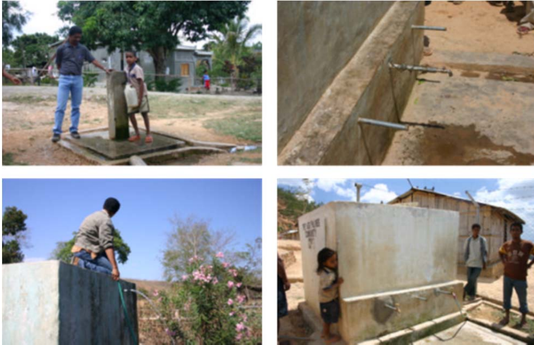
Pictures above: Examples of combination drinking water reservoirs and tap stands for bridging short periods with absence of water (LGSP), which are at present not widely used and tested.
