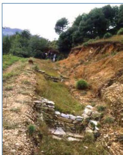
Picture left and drawing below: Erosion protection measures based on bio-engineering; small rip raps and vegetation.
